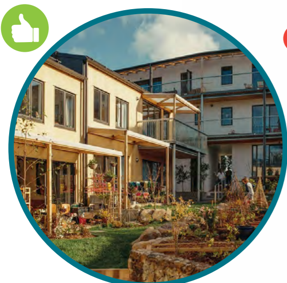
Co-Haus, Grey Lynn. Dwellings are orientated towards a communal open space creating a safe, well used area that fosters a positive sense of community for residents.
