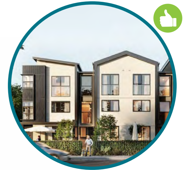
Karaka Grove, Takapuna. Use of different roof shapes to individualise each unit.
