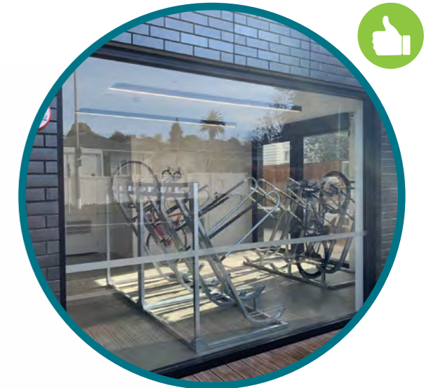
Modal, Mt Albert. Resident's cycle parking has been incorporated securely into the building facade with convenient access from the adjacent street.
