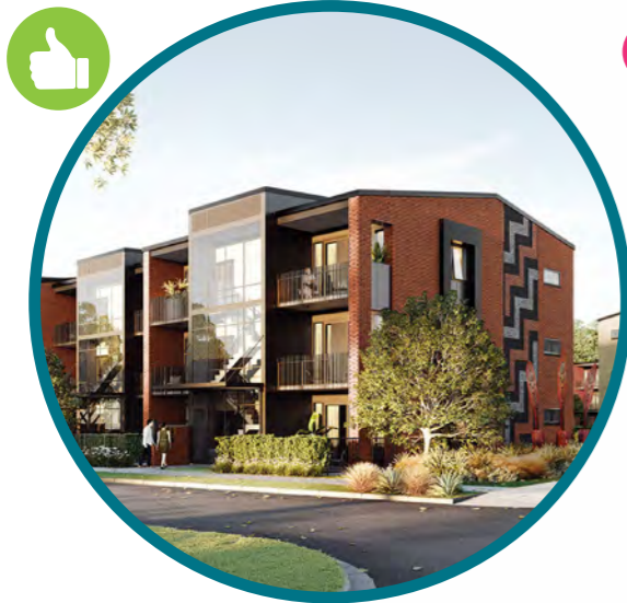
Northcote Development, Auckland. An example of using material to create façade articulation
