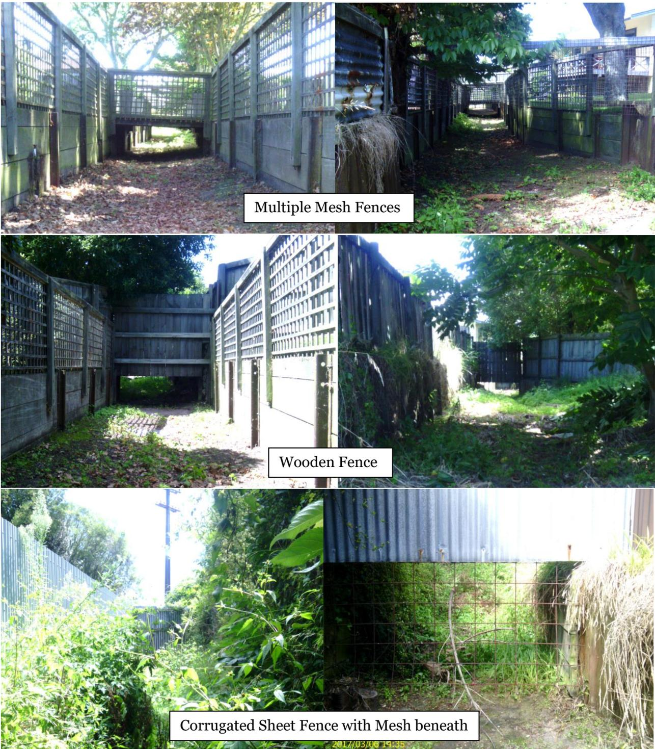
Figure 9-5: Potential Flow Restrictions in Timber-Lined Section
