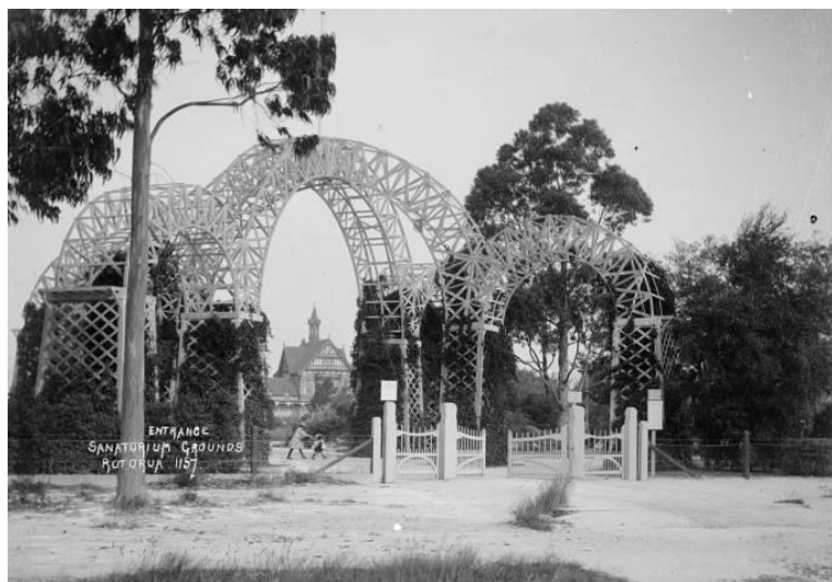
The Totara arches at the intersection of Hinemoa Street and Fenton Street were built for the visit of the Duke and Duchess of Cornwall and York to Rotorua in 1901. The latted timber frame held greenery and electric lights. The arches were designed to represent a crown. The structure was dismantled and re-erected at the entrance to the Government Gardens after the visit was over. It was threatened with demolition in 1974.
