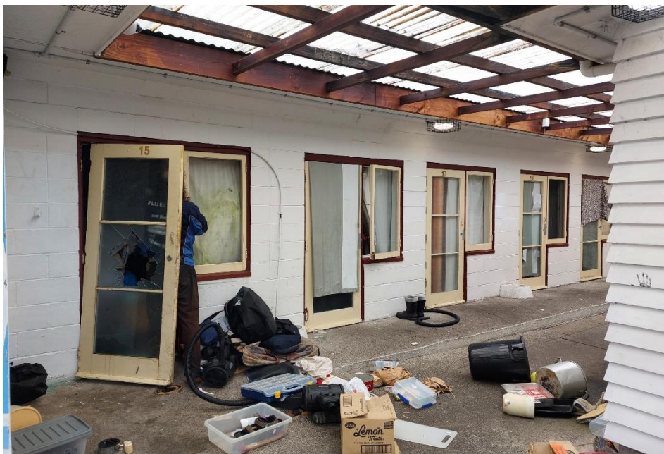
Image 4: Outside rooms 15, 16 and 17.
