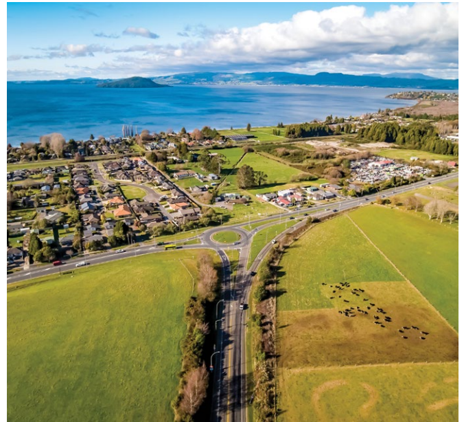
SH5/SH36 Ngongotahā roundabout
