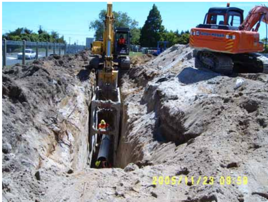
Sewer pipeline installation
