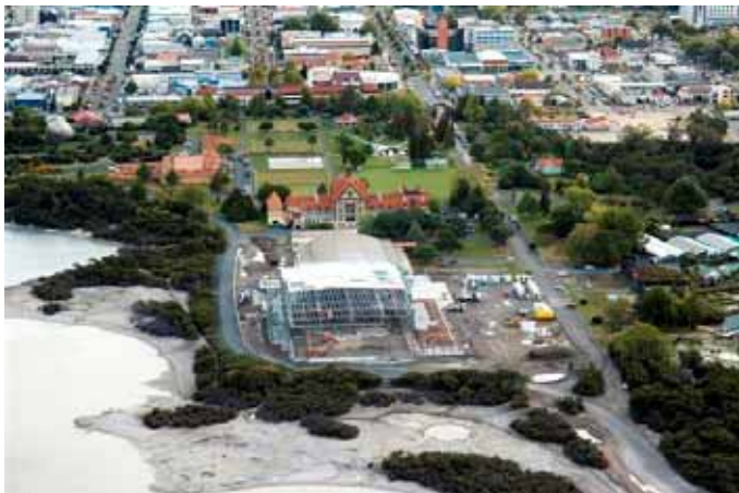
Aerial view of Energy Events Centre under construction
