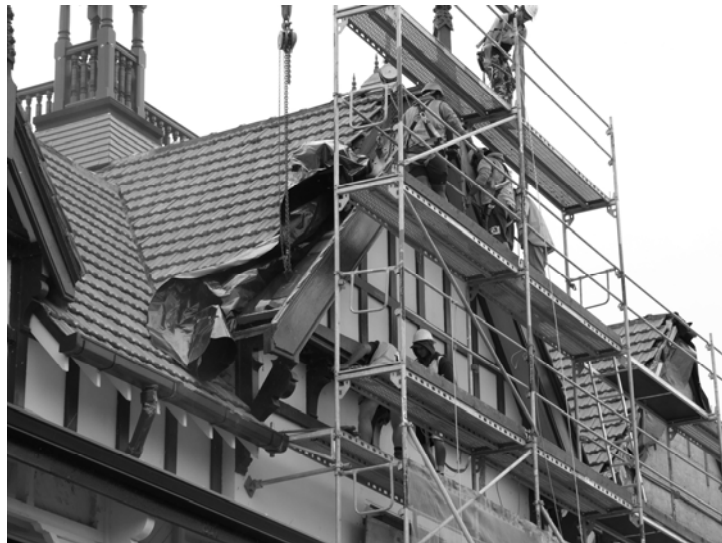
Construction work during the Rotorua Museum Centennial Project
