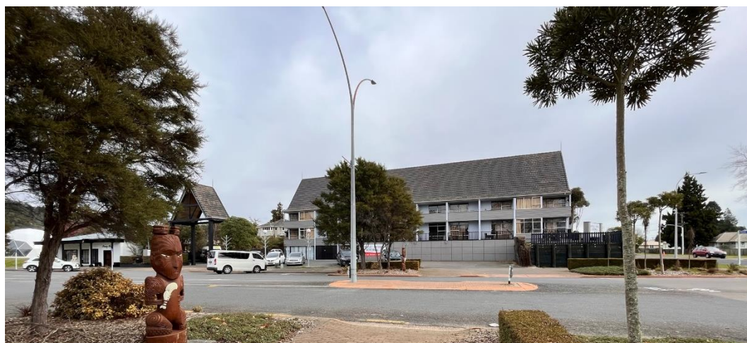
Figure 1: 7 Tryon Street (as viewed from Tryon Street)
