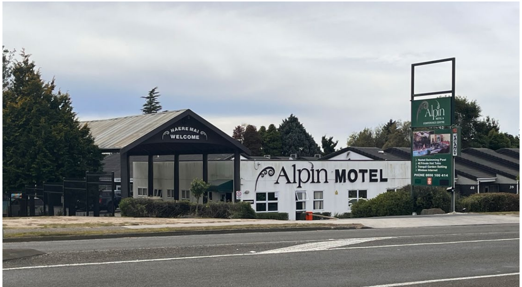
Figure 1: 16 Sala Street (as viewed from Sala Street)
