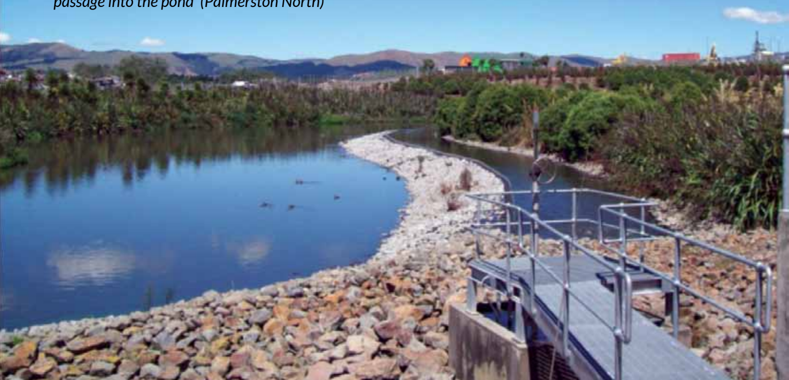
Wetland pond showing land (gravel/rock) passage into the pond (Palmerston North)
