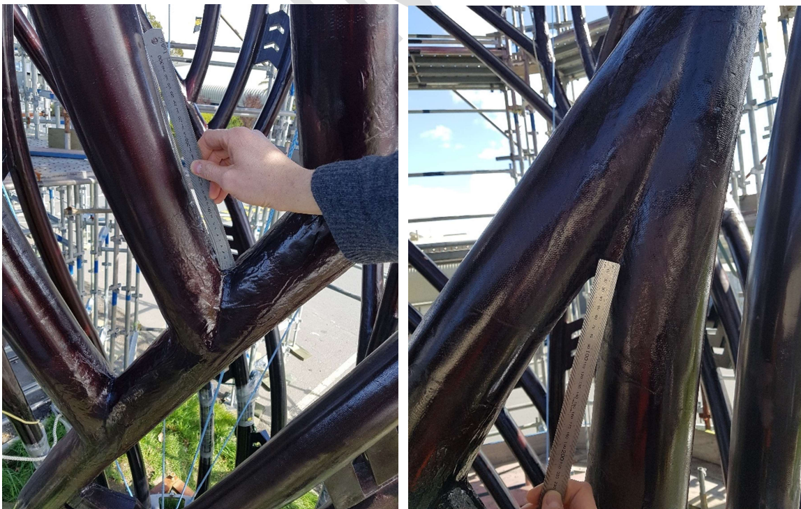
Figure 2. Example of inner tube connection taping checks
