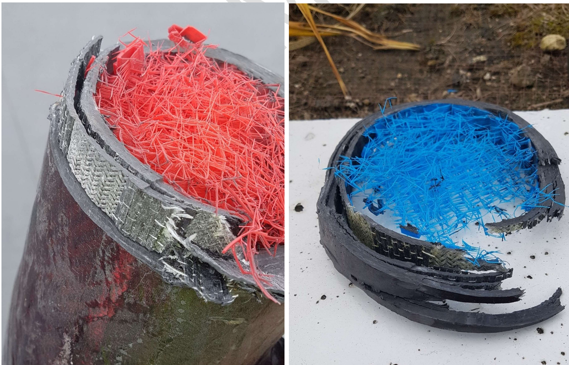
Figure 6. Inner tube sections removed during installation showing dry layers and interlaminar fractures/delamination
