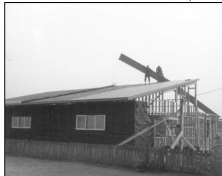
Construction of new hall, 1985
