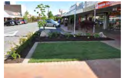
Pukuatua Street intersection upgrade
