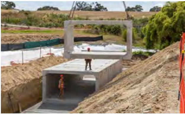
FIG. 5 Place first culvert into required position
