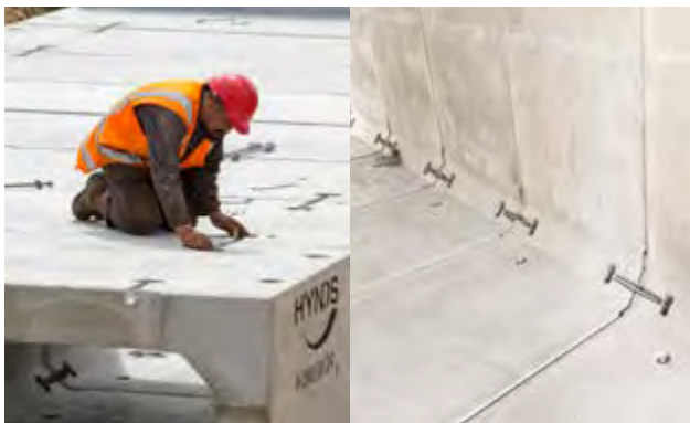
FIG. 7 Place threaded rod connecting set in groove. Tighten nuts equally at each end, using a socket wrench to a maximum torque of: Ø16 set: 100 Nm; Ø20 set: 125 Nm; Ø24 set: 150 Nm
