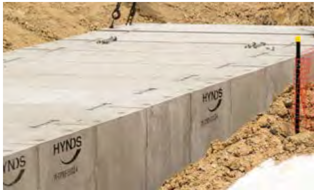
FIG. 8 Fill recess with Sikagrout 212 or equivalent.
