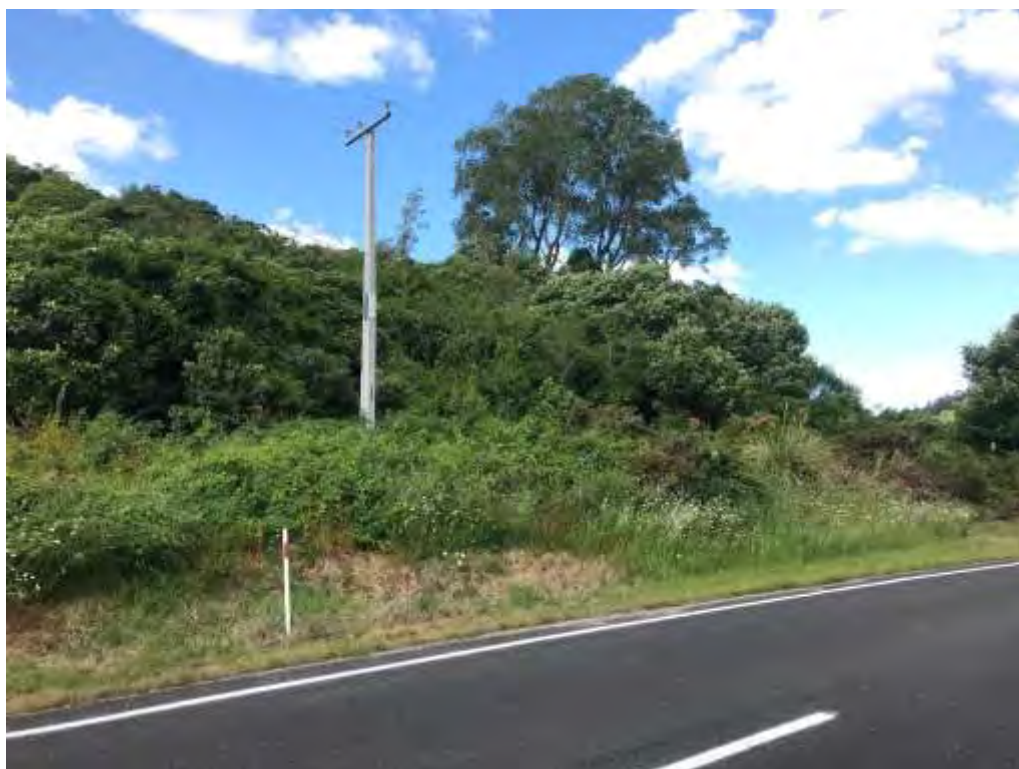
Plate 7: A recently-cleared access track along the power lines beside Tarawera Road. 26 November 2021.
