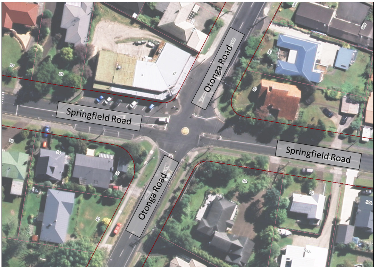
Figure 1-1 Springfield Road / Otonga Road Intersection
