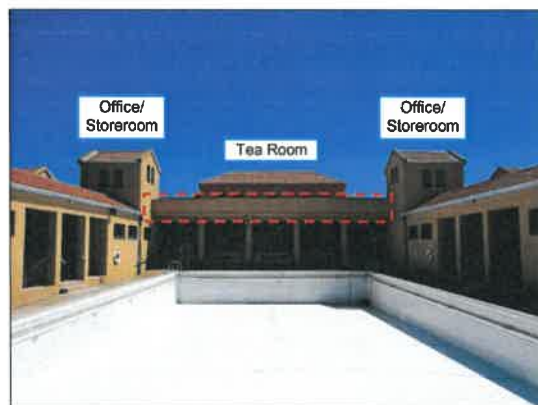
(f) Overview of the courtyard with offices, tea room and parapet
