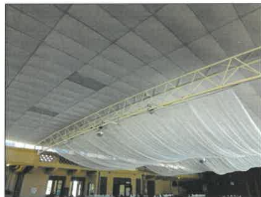
(l) New CHS steel truss
