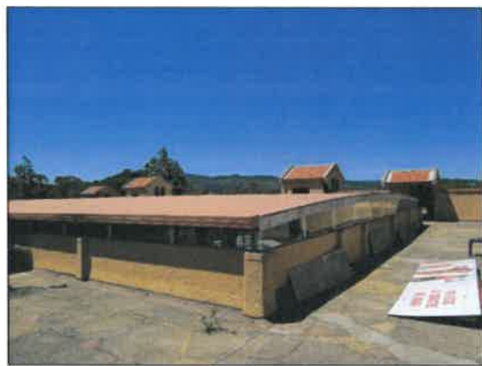
(d) Courtyard roof structure view from first floor
