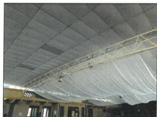
(l) New CHS steel truss
