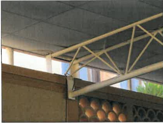
(m) Steel truss connection
