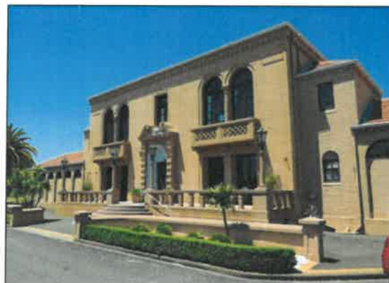
(b) North western elevation
