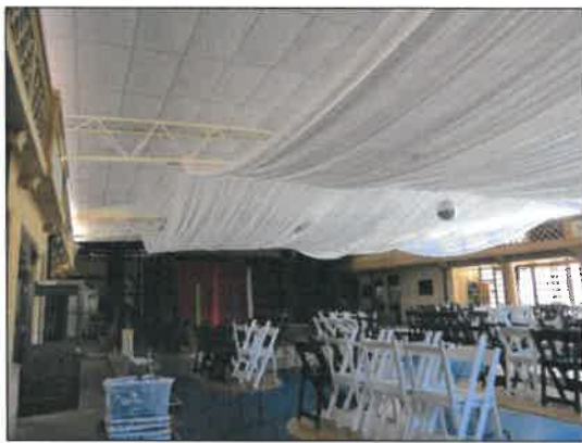
(c) Addition of roof structure to the courtyard which previously was the main pool
