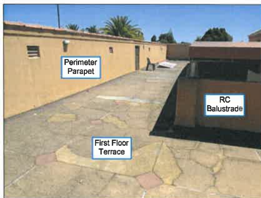
(e) The terrace and the parapet on the first floor
