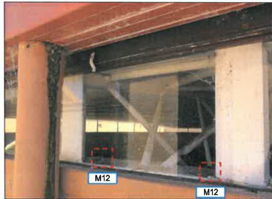
(n) Steel truss connected to RC balustrades by 2-M12
