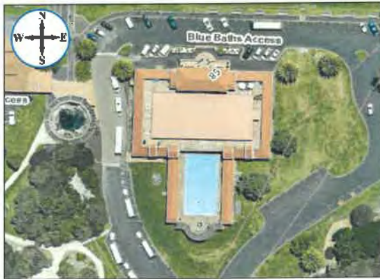
(a) Aerial view
