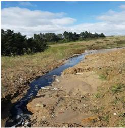
31. The bund of pond 2 (which is in the north-eastern corner of Stage 6b) had also been breached and leachate from pond 2 was overflowing at a high rate into an open stormwater drain. At the time, the officer thought that this open drain led to the leachate system but later that day she was advised that the drain actually flowed to stormwater pond B.
