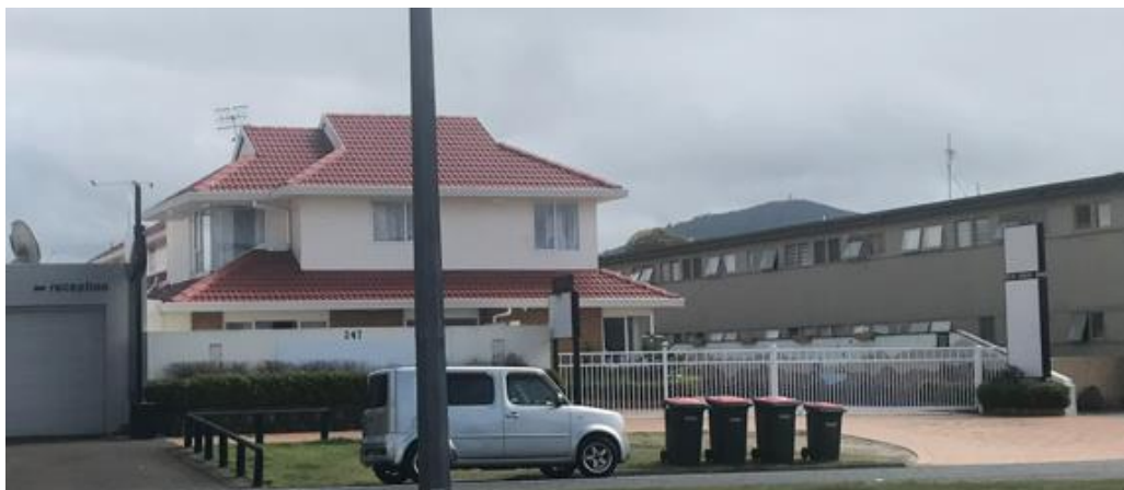
Figure 1: 274 Fenton Street & 12 Toko Street (as viewed from Fenton Street)
