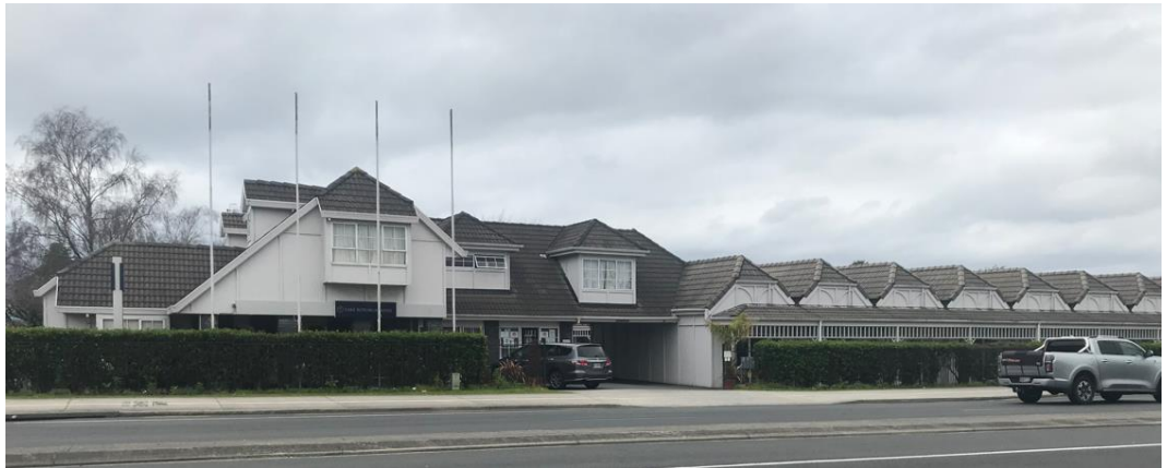
Figure 1: 131 Lake Road (as viewed from Lake Road)
