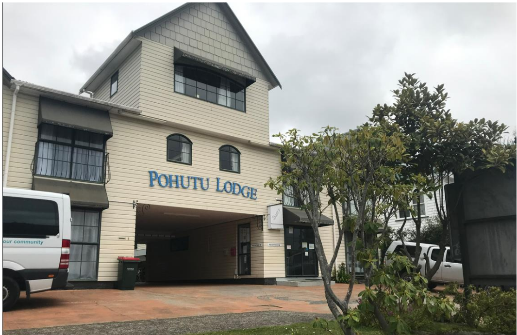
Figure 1: 3 Meade Street (as viewed from Meade Street)
