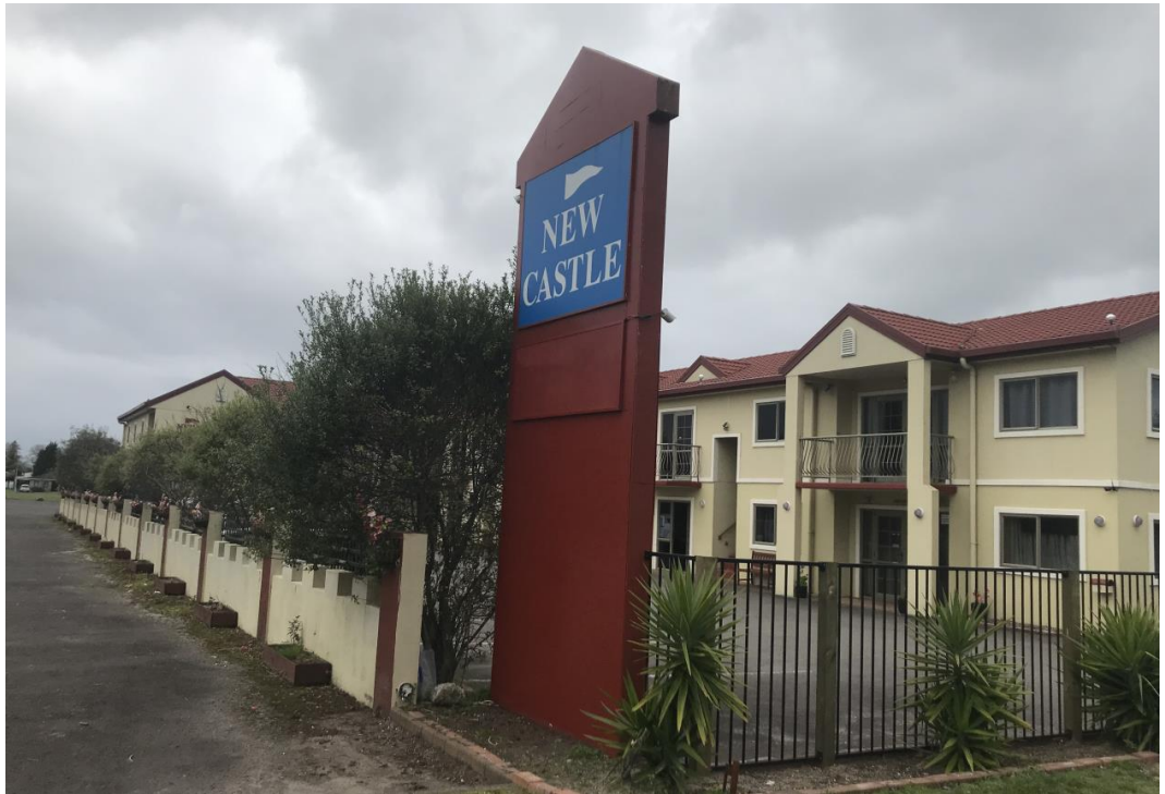
Figure 1: 18 Ward Avenue (as viewed from Ward Avenue)
