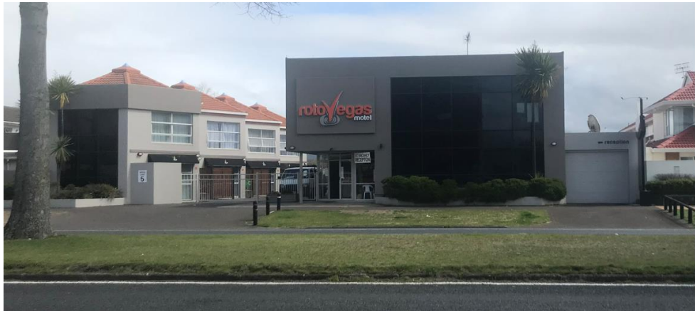
Figure 1: 249-251 Fenton Street/14-16 Toko Street (as viewed from Fenton Street)
