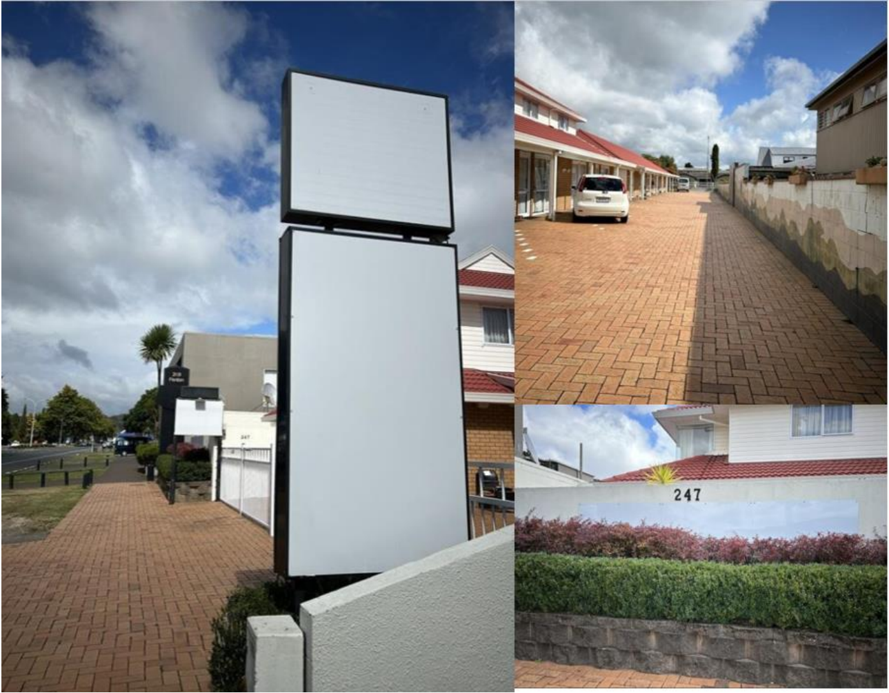
Figure 5-2 Ascot motel site visit photos
