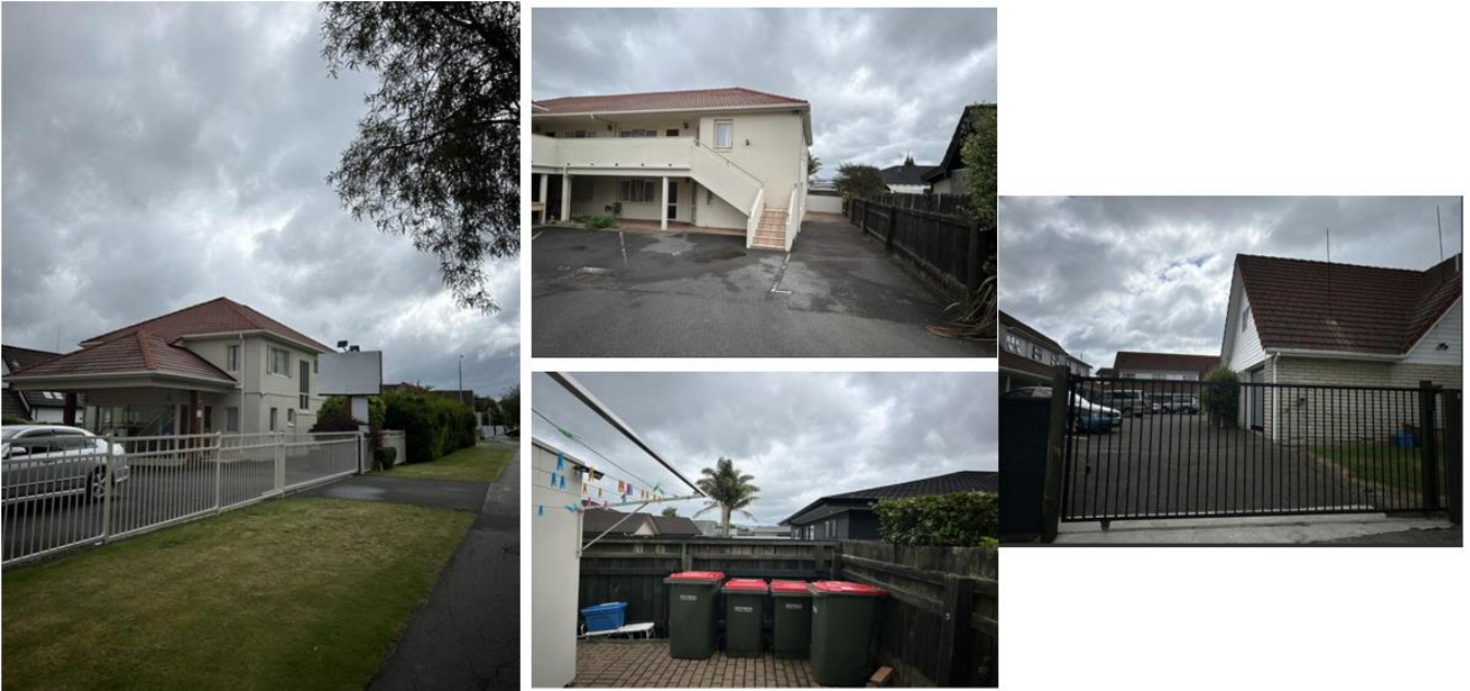
Figure 5-5: Geneva motel site visit photos
