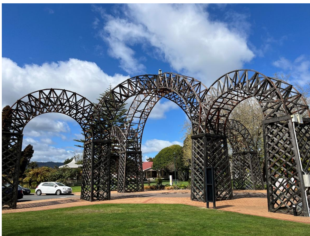
Figure 2: View of overall Structure (Looking to the South)
