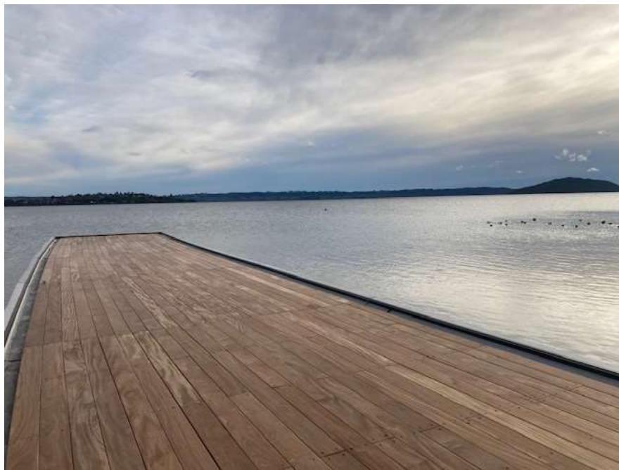
Stage 5 lake edge landscaping (top left), connection between boardwalks (top right) and new boardwalk (bottom)
