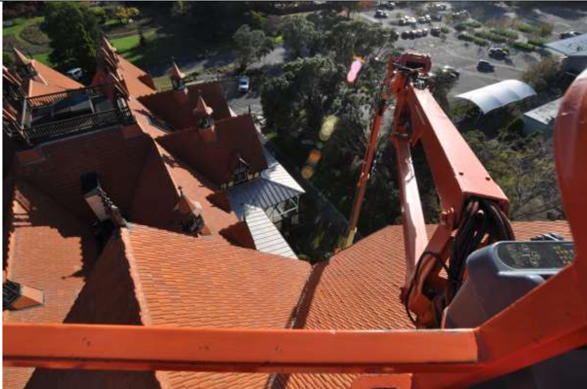
Roof inspections by EWP
