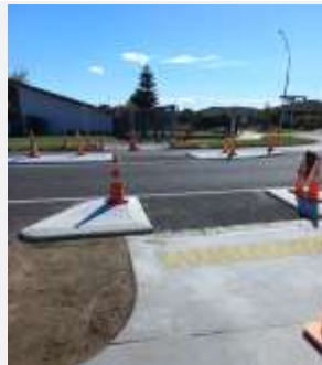
Vaughan Road shared path crossing
