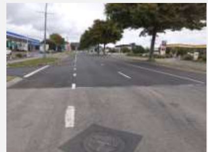
Yearly resealing (near completion (70%))
