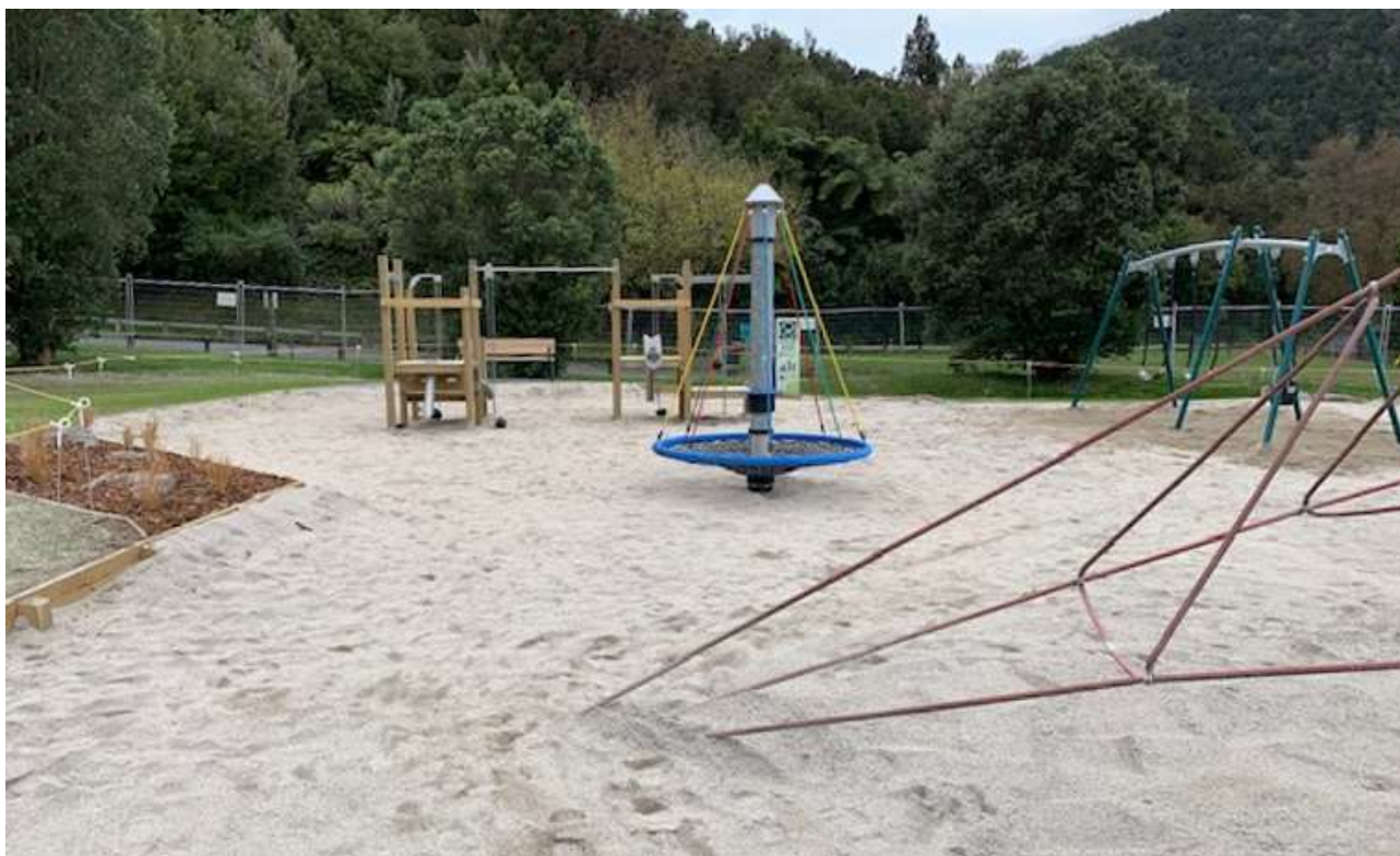
Tikitapu Playground renewal nearing completion
