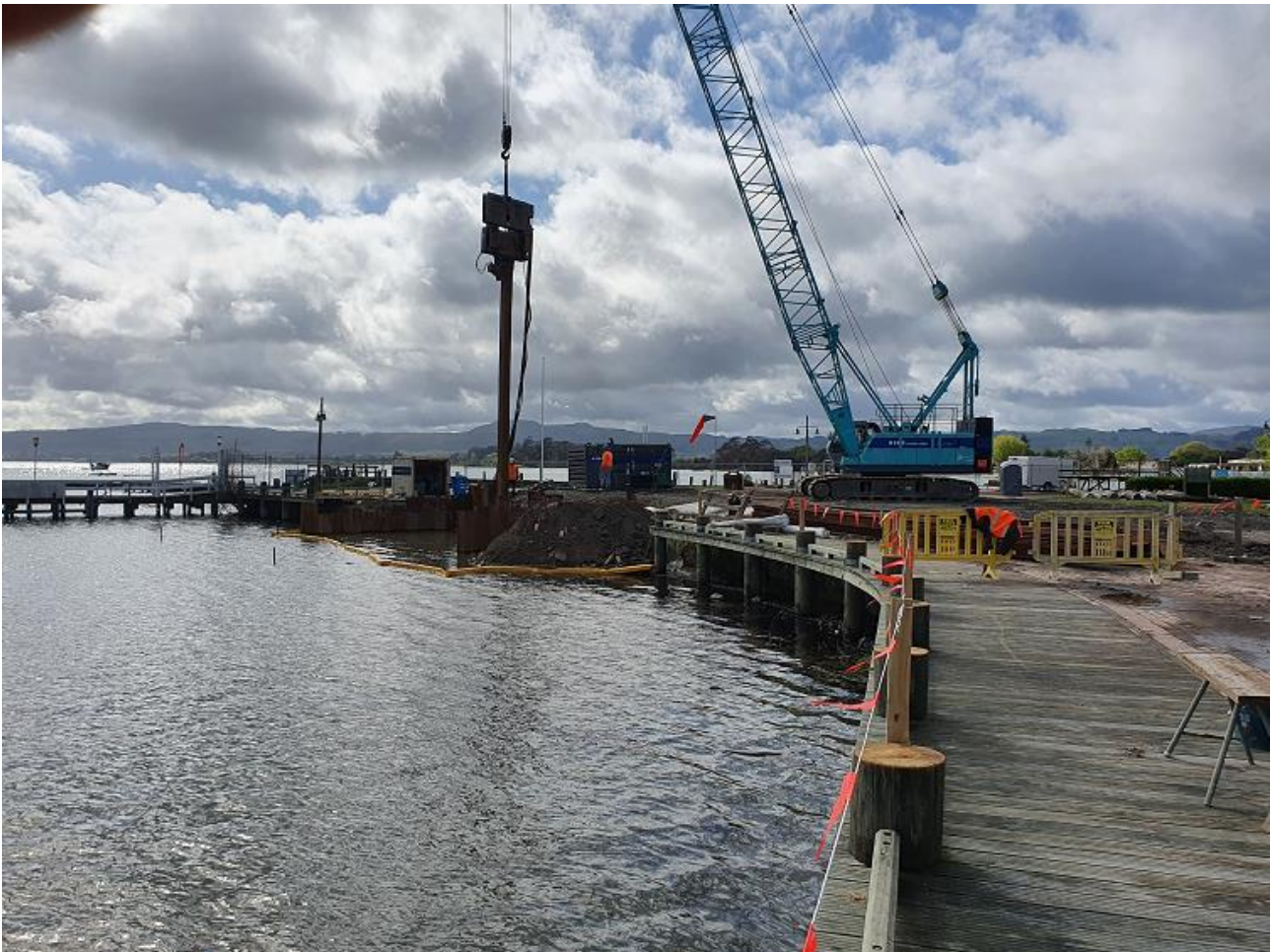
Stage 5 sheet piling beginning for the area for the western boardwalk
