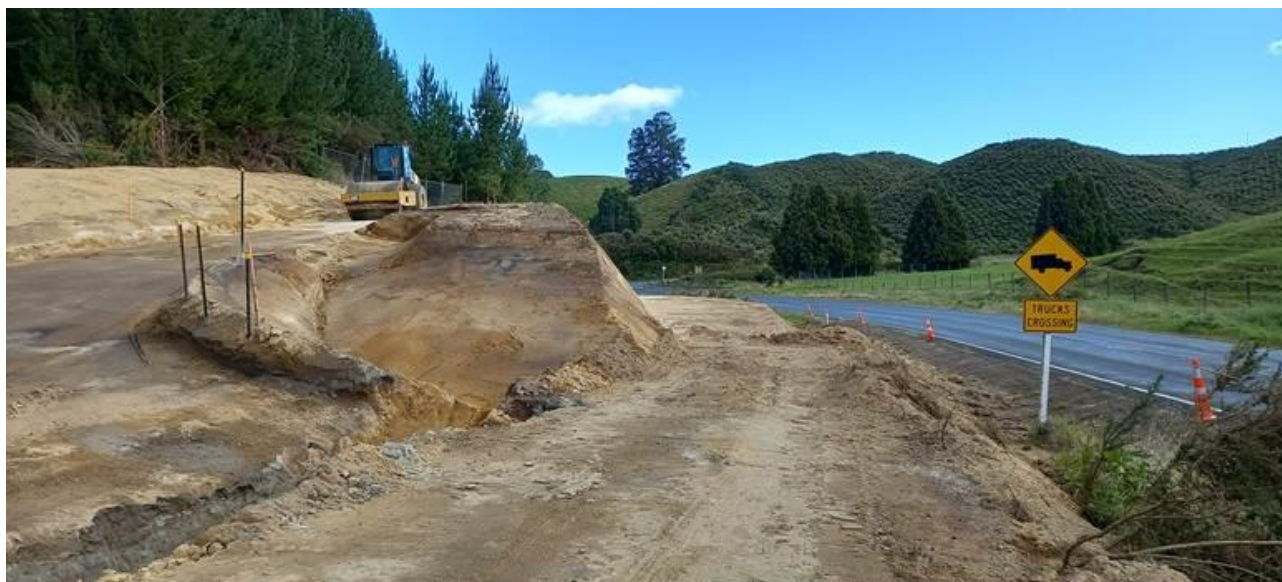
Photo: New Whakarewarewa forestry access road being created off Tarawera Road
