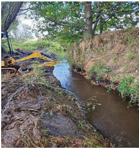
Photo: During the clearing
