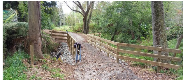
Photo: New culvert along Puarenga Stream
