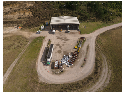
Transfer Station at top of landfill
