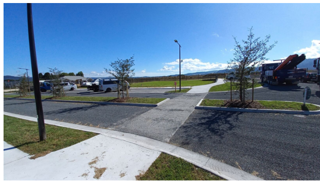
Manawa Gardens Development, Wharenui Road - new roads and infrastructure
