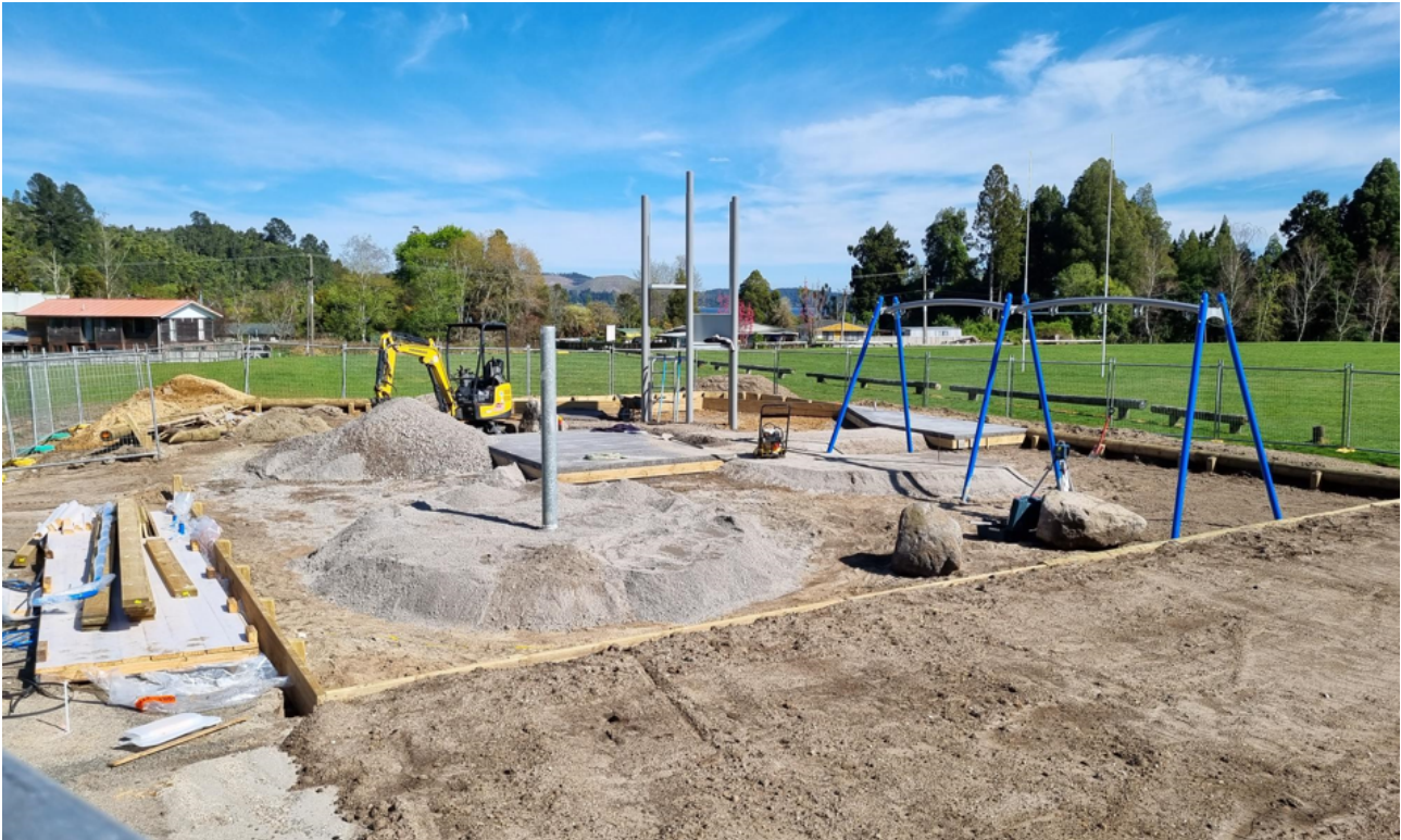
Haumingi Playground at Lake Rotoiti under construction.
