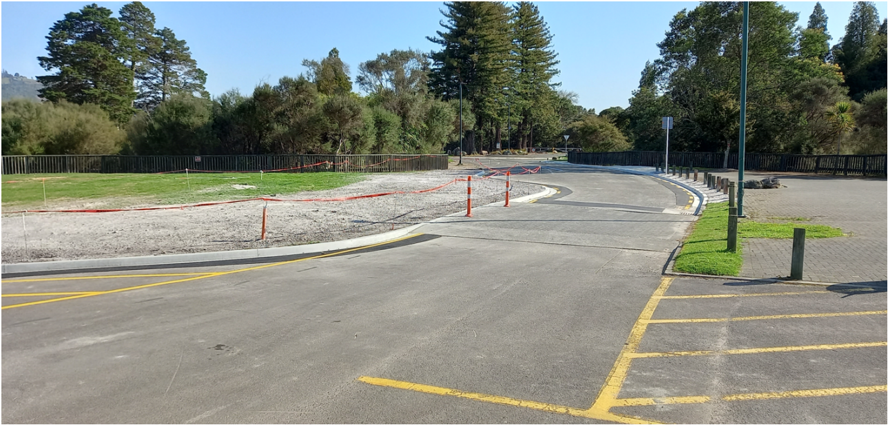
Realigned road pavement works completed on Kuirau Street
