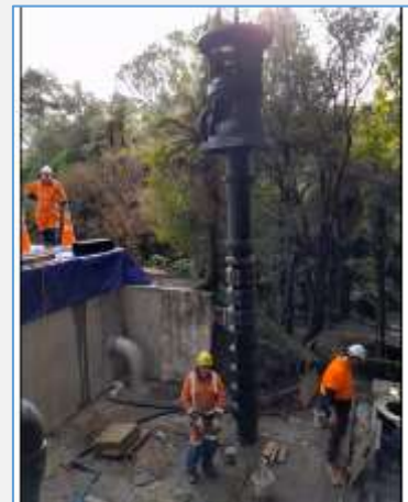
Taniwha Springs pump removal
