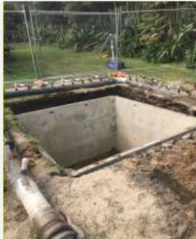
Rotoiti Sewerage Scheme - typical trench shield and dewatering system in place
