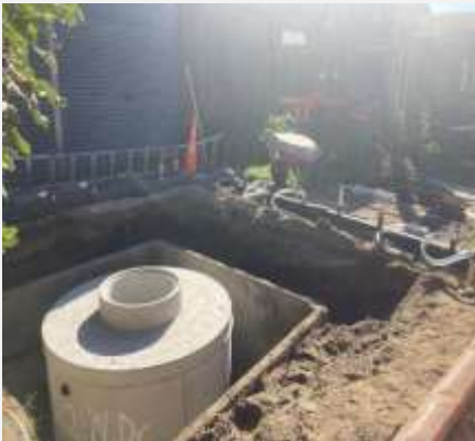
Rotoiti Sewerage Scheme - tank install on Wharetoroa Dr
