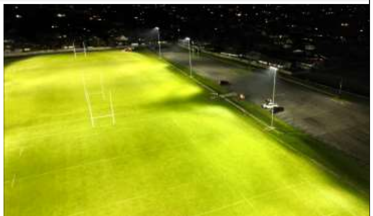
Above: Sports field lights installed for Westbrook 1 and 2 fields
