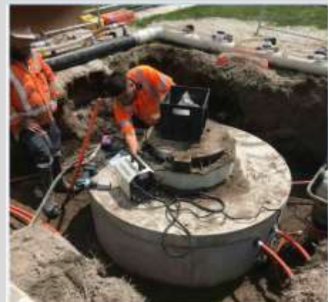
Biolytix system being installed
