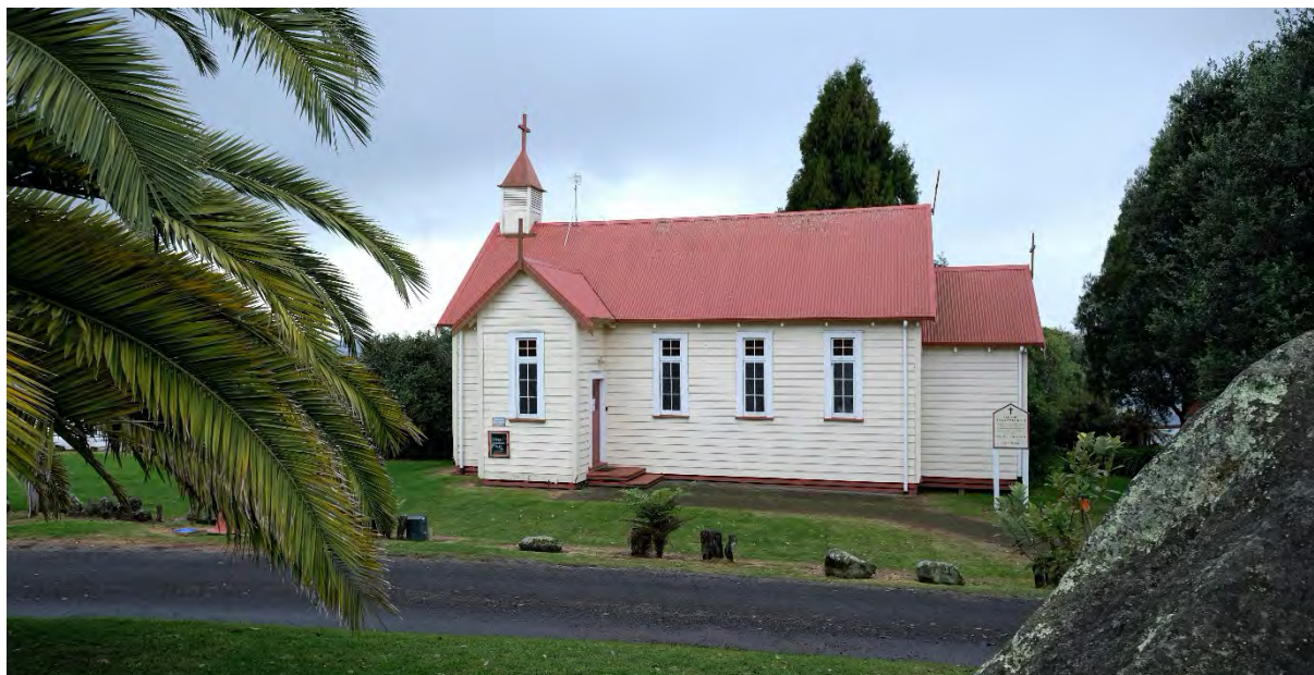
Figure 4 St Peter's Anglican Church, looking north. SRA 2022
