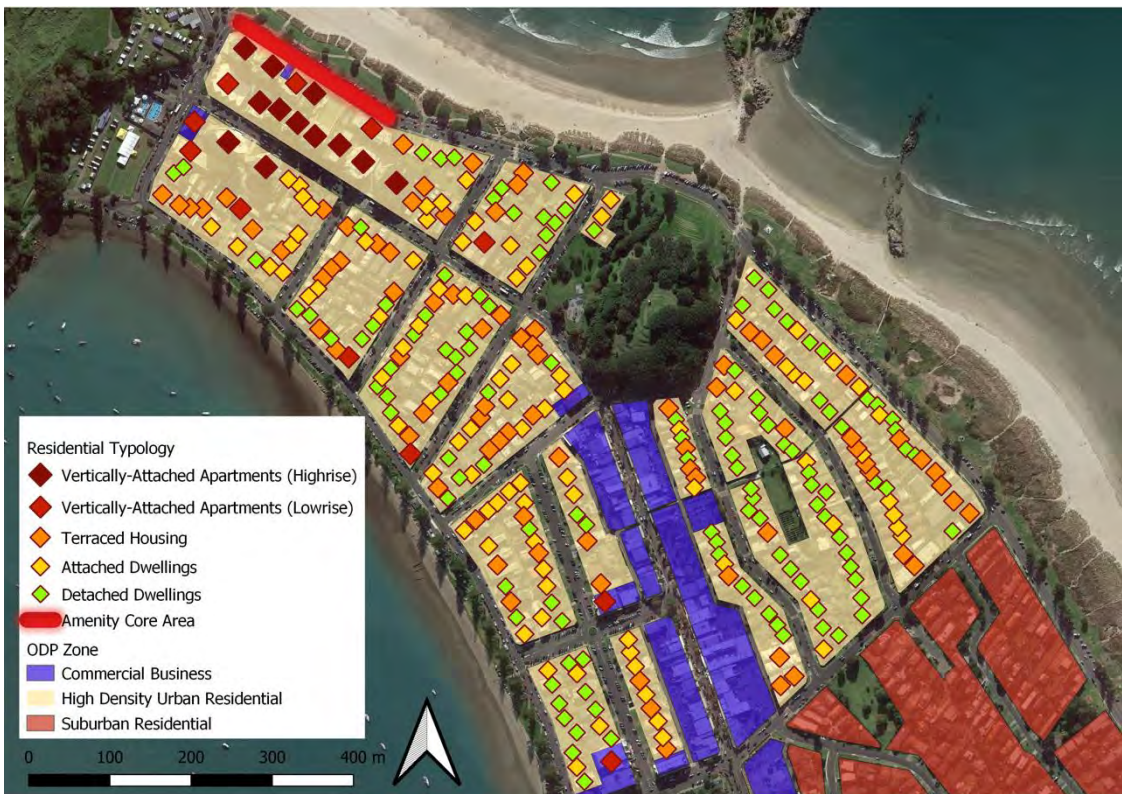
Figure 4-6: Residential Development Patterns by Typology in Mt Maunganui's High Density Urban Residential Zone
