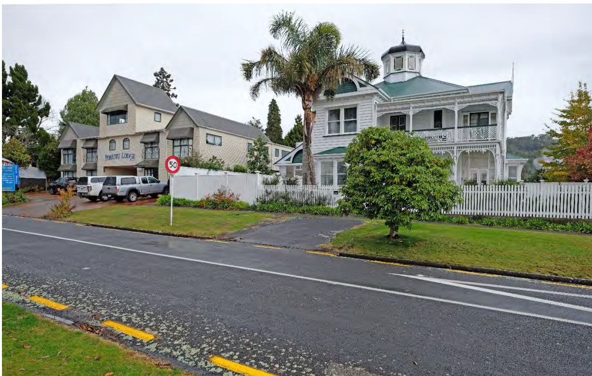
Figure 8 1 Meade Street ( Landmark Restaurant ) from cnr of Fenton & Meade Streets. SRA 2022
