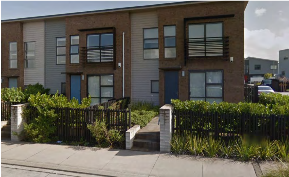
Figure 3 – Low street fencing on a medium density development (Hobsonville, Auckland)
