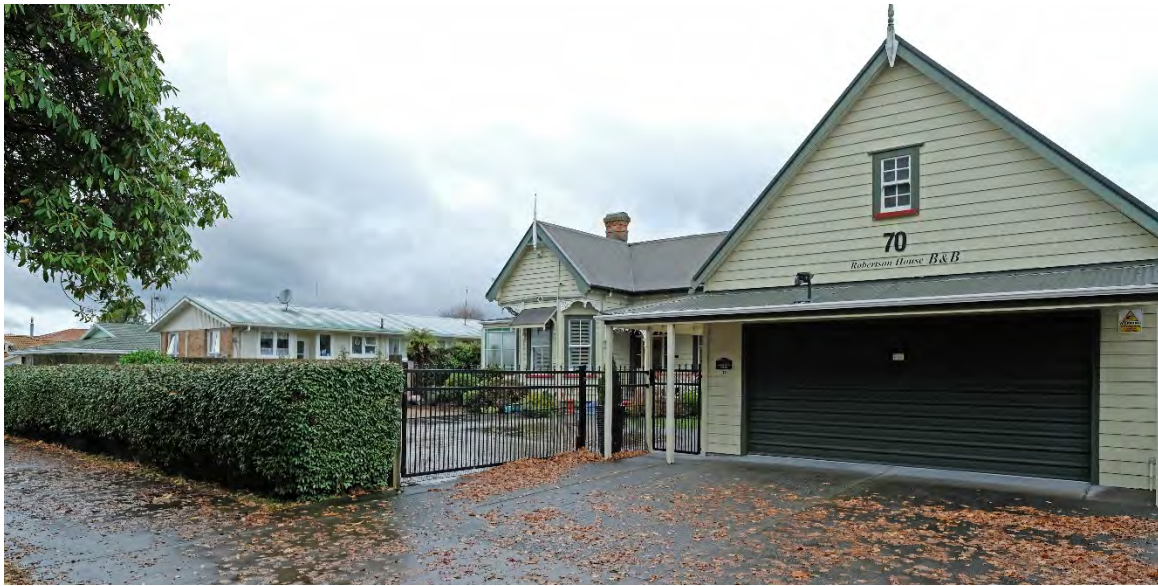
Figure 2 Robertson House, 70 Pererika Street looking southeast. SRA 2022
