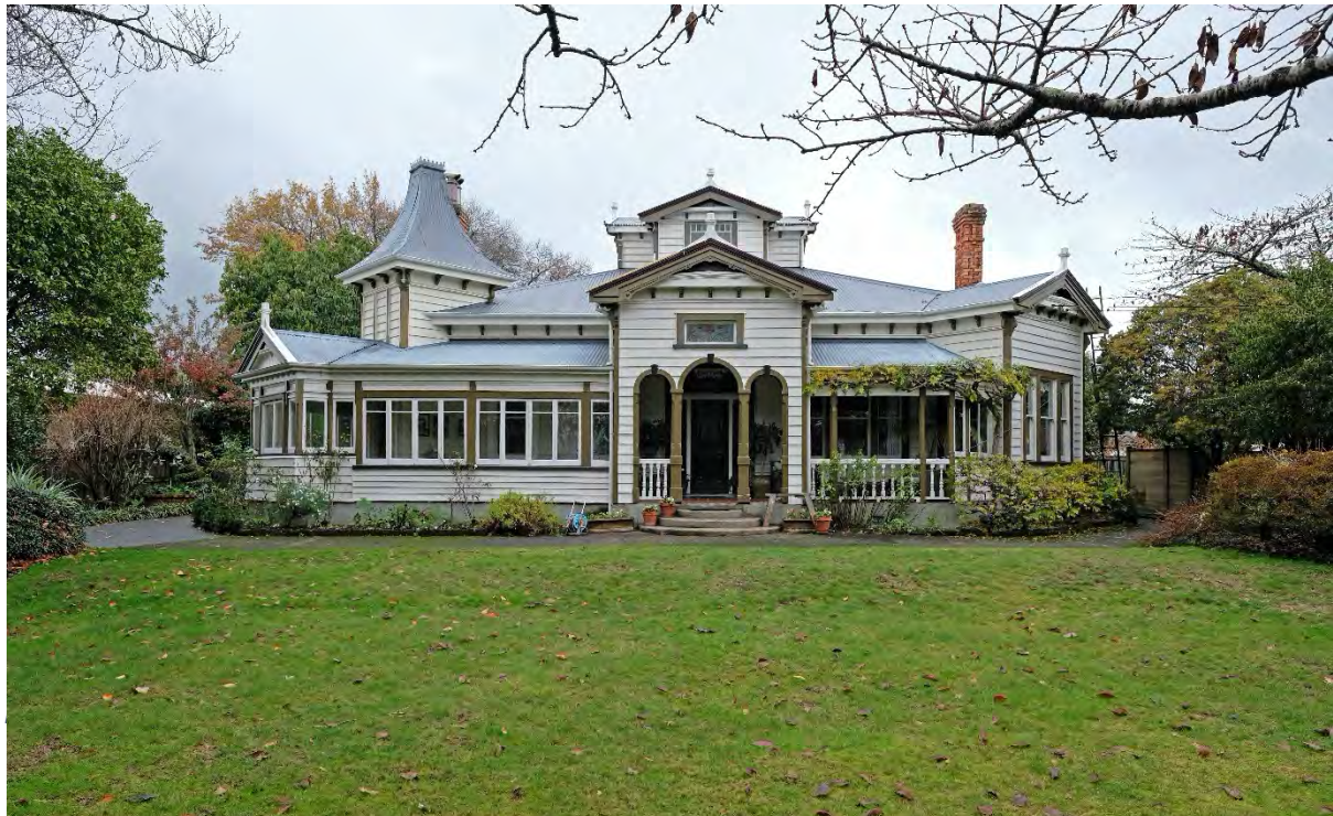
Figure 4 63 Miller Street original front elevation, looking south. SRA 2022
