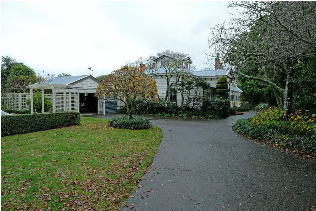
Figure 2 63 Miller Street from top end of driveway, looking northwest. SRA 2022
