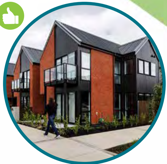
Buckley Terraces, Hobsonville. The internal layout and associated façades have been designed to address both street frontages.
