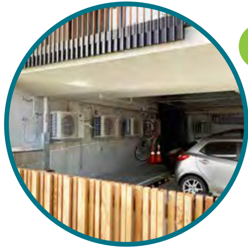
Air conditioning units have been incorporated into an undercroft parking area away from the street frontage avoiding unnecessary visual clutter.
